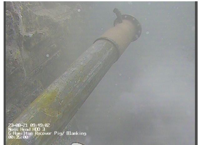
Photo of the HDD3 exit point showing the protruding duct
